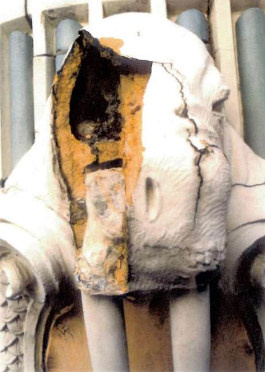
Figure 2: Fractured terra cotta walrus head. Note the degree to which the grout fills the terra cotta void. Credit: Wiss, Janney, Elstner, 1995
