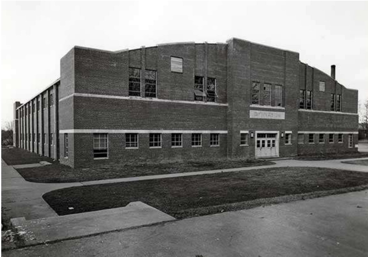
Figure 9: The Gym at Elon University is a typical example of Gym D construction with concrete structural walls, brick, and stone facing.
