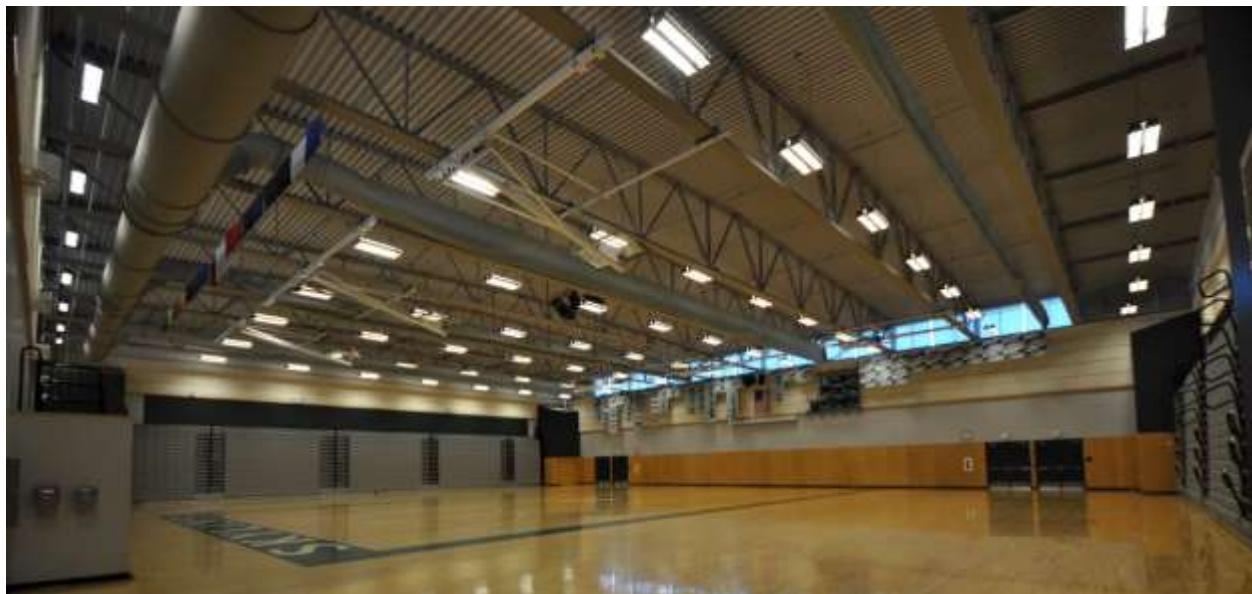
Figure 6: The gym at Skyline High School in Issaquah, WA, is an example of the metal framed roof structure in Gym B and C.
