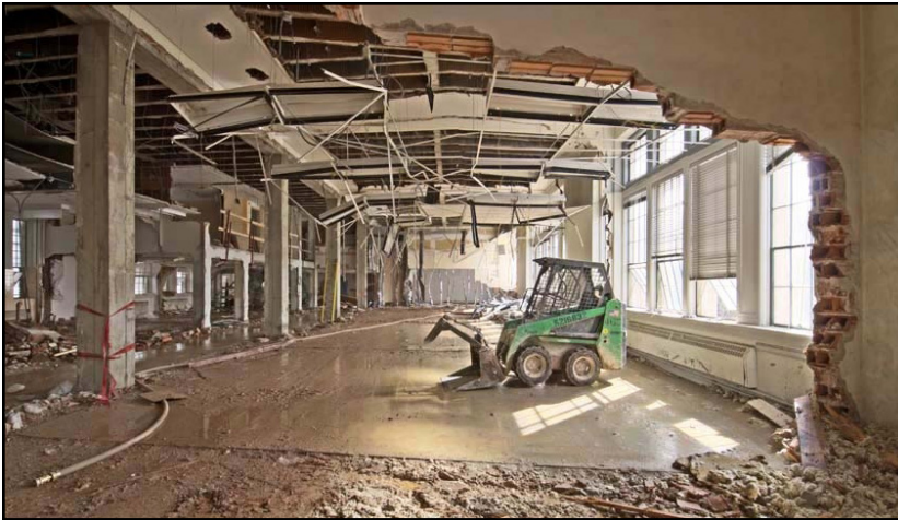
Figure 24: All interior construction was demolished to allow for new building systems. Credit: John Stamets, 2008, courtesy UW CPD.
