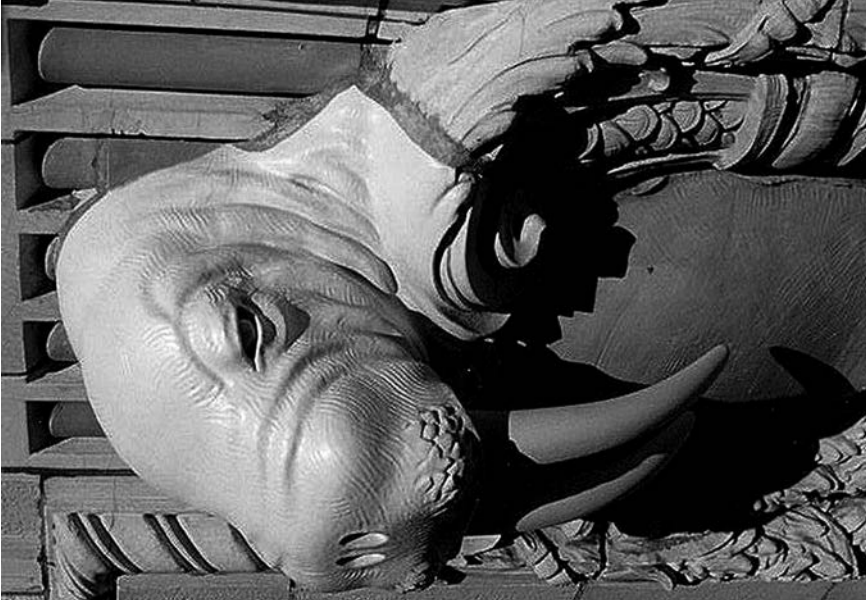
Fig. 8. 1996 replica walrus head. The joints between terra cotta pieces are filled with mortar after the epoxy sets around the threaded rod anchors. (Credit: Wiss, Janney, Elstner Associates, Inc.)
