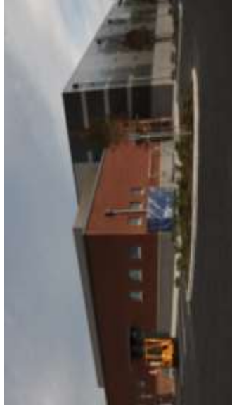
Figure 3: The Gym at Shorewood High school in Shoreline, WA is an example of Gym C construction. The main volume of the gym has CMU exterior walls and metal roof structure. Credit: Brian Rich, 2013.
