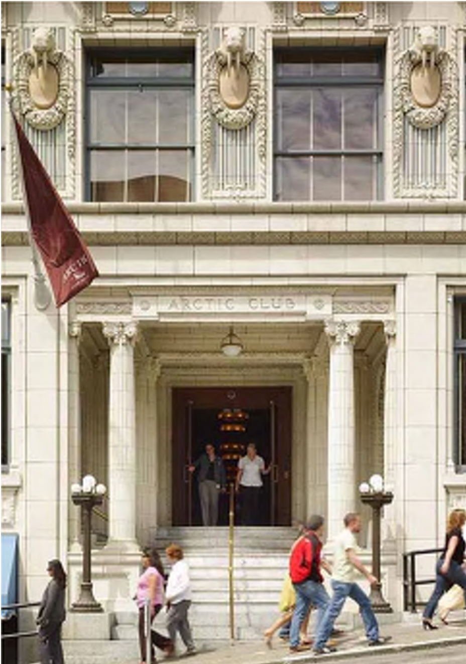
Figure 52: Cherry Street Entrance to the Arctic Hotel. Credit: Weaver Architects, 2005
