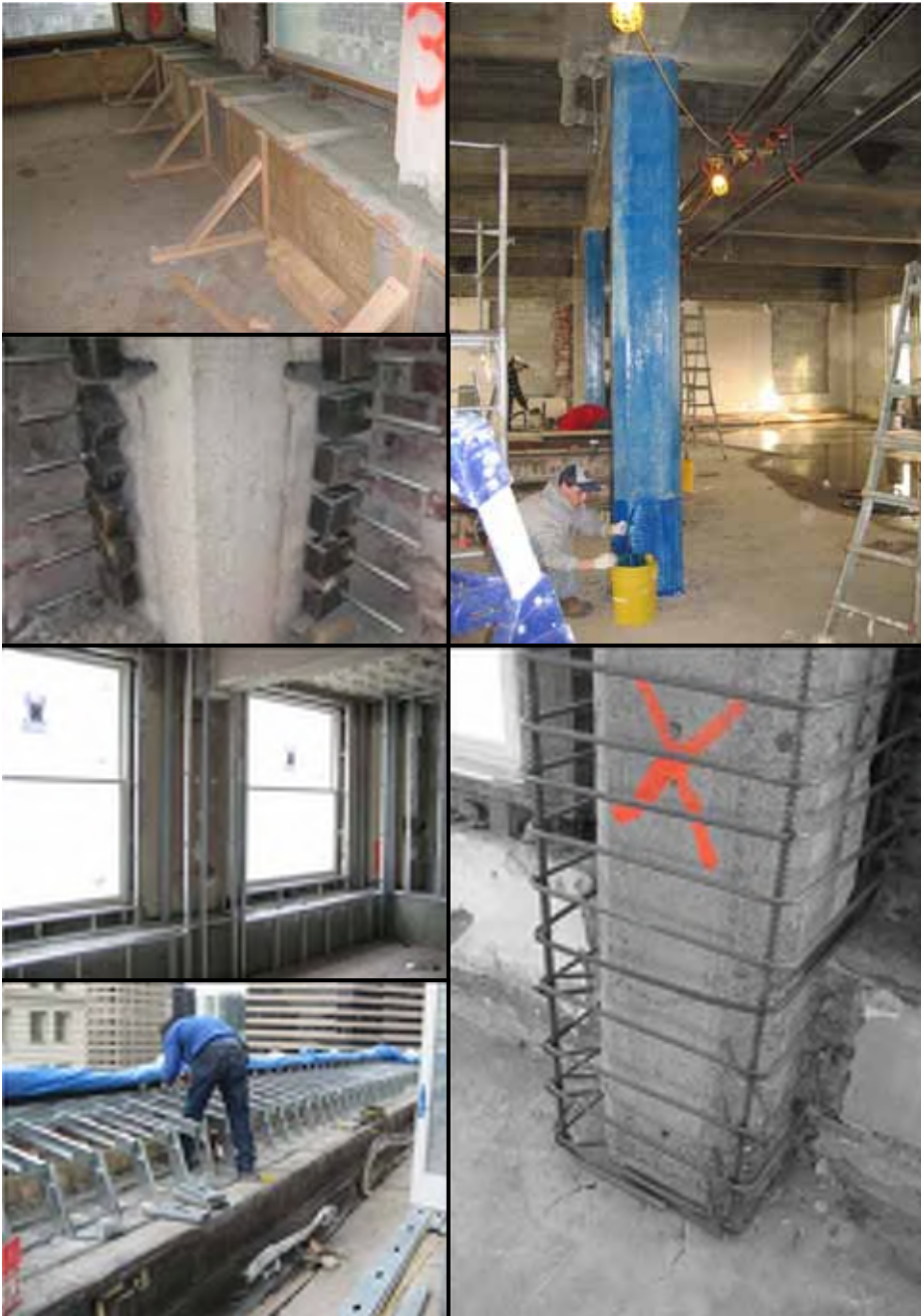
Figure 43: 2005 Rehabilitation of the Arctic Hotel. Credit: Weaver Architects, 2005.
