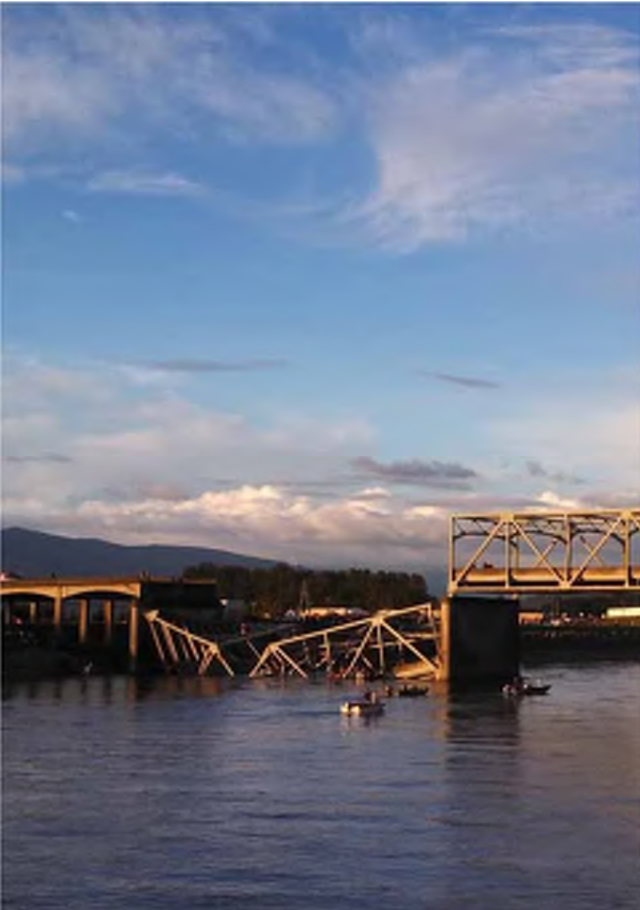
Figure 14: The collapsed I-5 bridge at the Skagit River was “functionally obsolete.” Credit: http://en.wikipedia.org/wiki/File:05-23-13_Skagit_Bridge_Collapse.jpg
