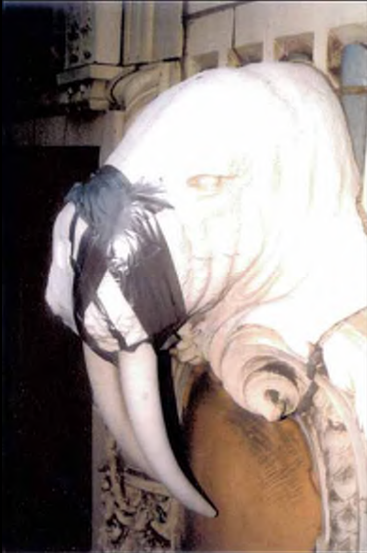
Figure 47: 1995 photo of the deteriorated walrus head at the Arctic Building. Credit: Wiss, Janney, Elstner, 1995.
