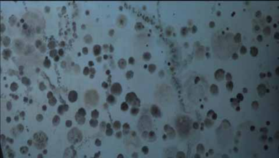
Figure 4: Mold caused by too much water vapor trapped within a building. Credit: http://media.kmvt.com/images/MOLD1.jpg_BIM.jpg
