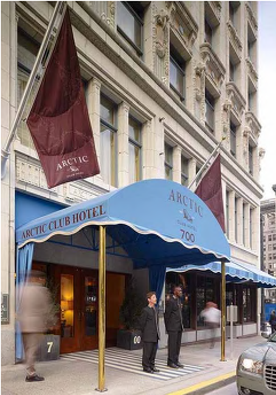
Figure 56: The Third Avenue Entrance to the Arctic Hotel after the 2005 rehabilitation. Credit: Weaver Architects, 2005.
