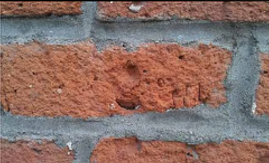
Figure 6: Sandblasted brick removes the fire skin from the brick. Credit: http://www.permies.com
