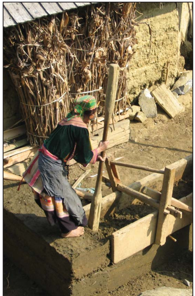
Figure 7: Rammed Earth house in Vietnam. Credit: http://en.wikipedia.org/wiki/Rammed_earth
