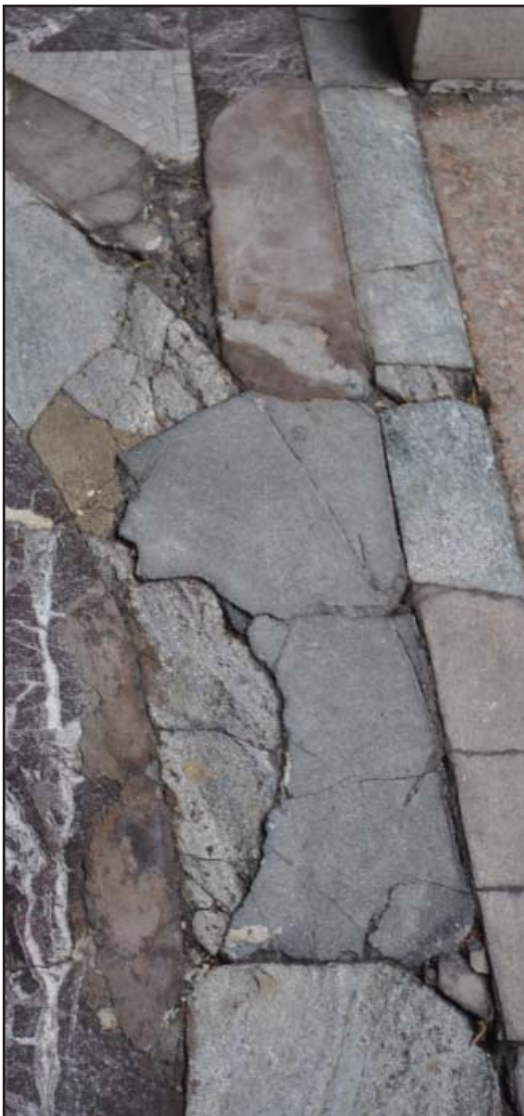
Figure 3: Stone floor at the chapel at Columbia University in 2013. The stone material is failing for obscure reasons, but was not a future-proof selection for this location. Credit: Brian Rich, 2013.
