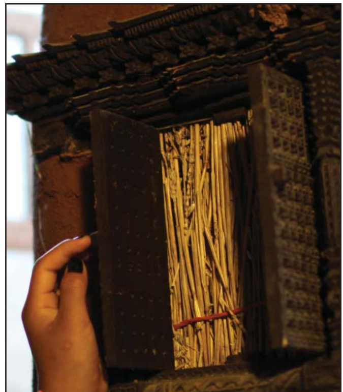
Figure 10: A straw window in the wall of a straw and adobe house. Credit: http://www.wabash.edu/photo_album/home.cfm?photo_id=18004&photo_album_id=2504
