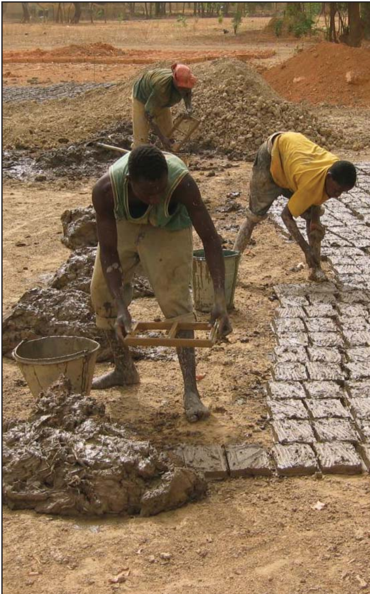
Figure 11: Making mud bricks in Africa. Credit: http://www.lavoutenubienne.org/sites/default/files/stock/photos/technique/bricks.jpg
